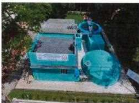
360 KLD STP at General Hospital, Thrissur
