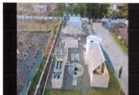
1 MLD CSTP at Padanappalam, Kannur
