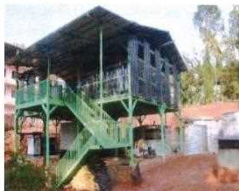
1 MLD STP at Kozhikode medical College
